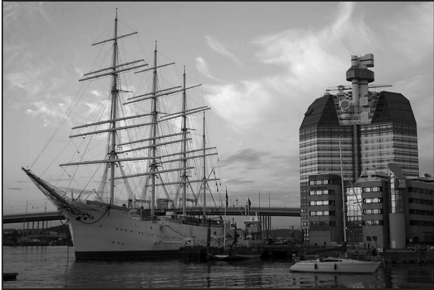
Figure 1.1: The improvised headquarters for the emergency response team is located in the high “Lipstick” building in Gothenburg, at the shore of Göta Älv. Photo, Painting the sky with lipstick , by Jonas Ahrentorp.
